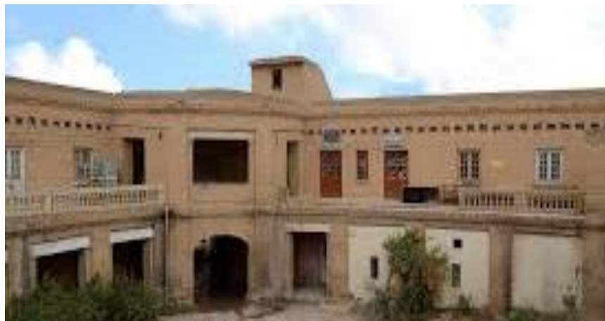
Figure 8. Al- Saraai Structure
