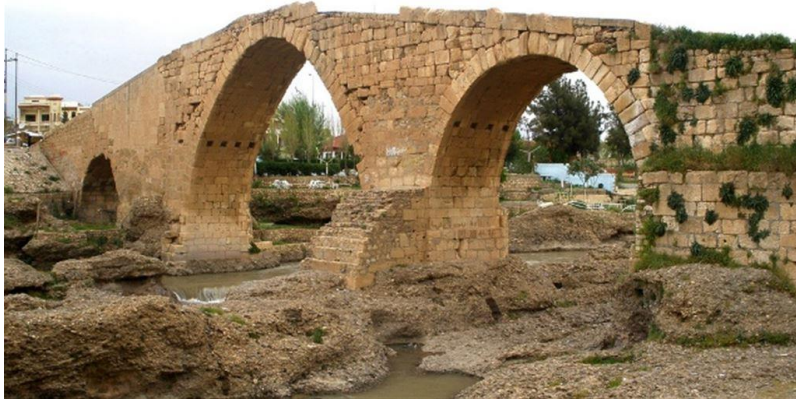
Figure 5. Historic Buhrez Arcade
